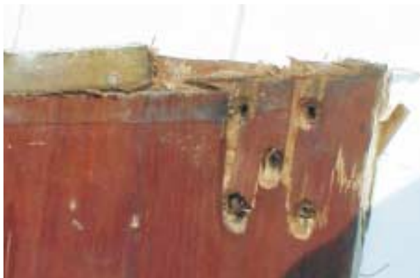
Below—Two views of the starboard bulkhead where the chainplate let go shows the result of accumulated water damage and heavy loads.
