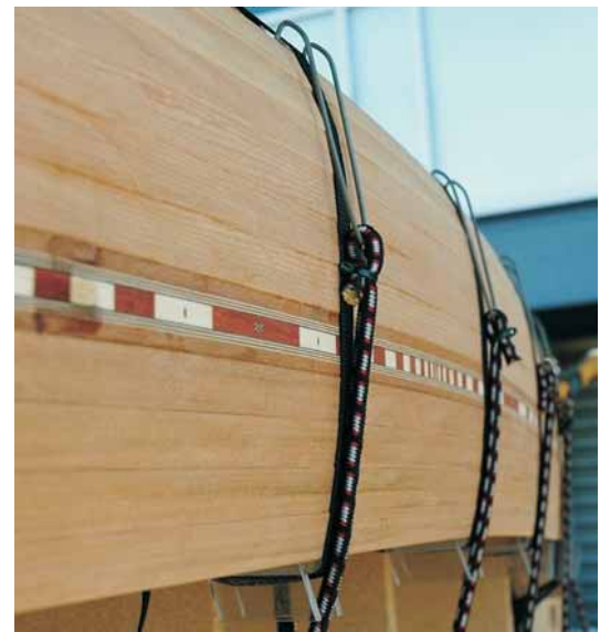
Below —The alternative strip building technique in use.
