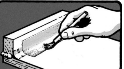
The fiberglass tape can be used to patch cracks and holes, or provide abrasion resistance to wear points such as stems and keels or the edges of paddle blades and centerboards.
