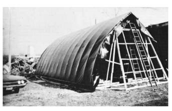
Figure 8-17 Plastic covering stretched over framework.
