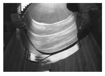
**Figure 2-4** The trimaran *Adrenalin's* hull is %'' (9.5mm) strip-planked cedar sheathed with unidirectional carbon fiber.
