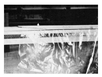
**Figure 12-5** Plastic sheeting woven back and forth between stringers contains the excess epoxy runout and prevents bonding of the stringers to each other. When placing this plastic sheet, avoid pinching the plastic in any of the scarf joints.
