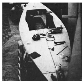
**Figure 27-32** The Luders 16 deck covered with <sup>1</sup>/<sub>4</sub>" (6mm) okoume plywood. The teak overlay will contribute to deck strength and stiffness.
