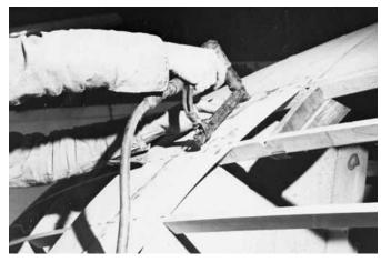
**Figure 22-14** Stapling the first layer of planking to the topsides. Note the laminated curved frame and blocking in the upper right as well as limber holes cut in stringers next to blocking.
