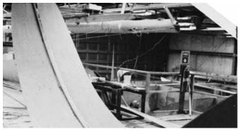
**Figure 25-3** Plywood panels and sheer clamps laminated to a large curve to help develop fullness in the upper sheer area of the completed hull.
