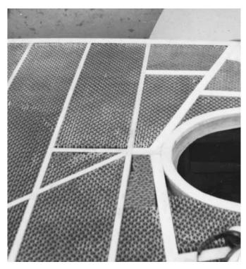
**Figure 11-14** A cored deck constructed using lightweight beams and resin-coated paper honeycomb core material. See Chapter 27 for a full description of this deck construction.
