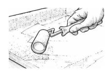
Figure A-29 Coat the surface to fill the weave before the wetout becomes tack free.
