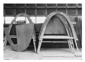
**Figure 17-10** Permanent frames ready for set-up. These frames have legs and spalls attached. They have been prefinished and notched for stringers.
