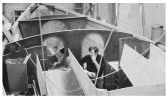
**Figure 27-13** An unusual slingshot-shaped cockpit is set in place on *Golden Dazy*. It is trued up with temporary bracing and blocking. Then the deck framework is installed around its perimeter.
