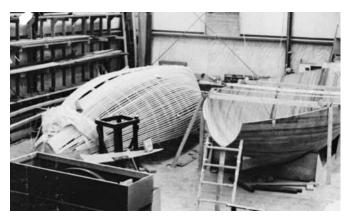
**Figure 21-25** The hull is in a cradle and immediately trued up with the waterlines. Temporary bracing at the sheer stabilizes the shape of the hull while interior joinery is installed. The ladder at the open transom provides easy access to the interior of the hull.
