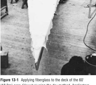
**Figure 13-1** Applying fiberglass to the deck of the 60' (18.2m) proa *Slingshot* using the dry method. Applicators have wet out the glass cloth around the daggerboard slot and are working toward the bow and stern.
