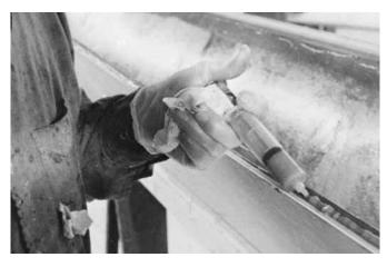
**Figure 11-19** A disposable syringe being used to apply a bead of thickened epoxy.
