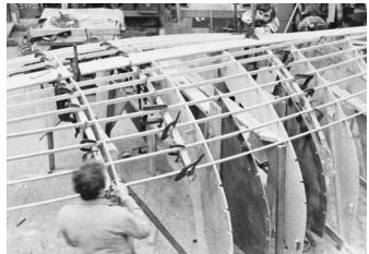
**Figure 22-11** Laminating floors over stringers. To ease the job of laminating and installing floor timbers, it was done before the topside stringers were installed.
